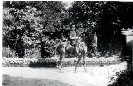
Figure 2.101 Correcting the major defects
